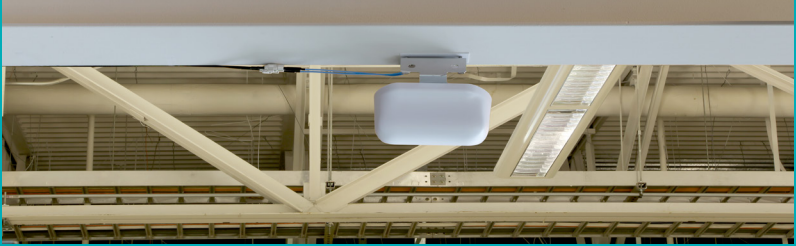
IN-BUILDING DAS ON I-BEAM
